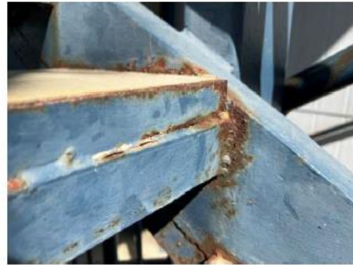
Photo 3 – Failing paint and corrosion.
