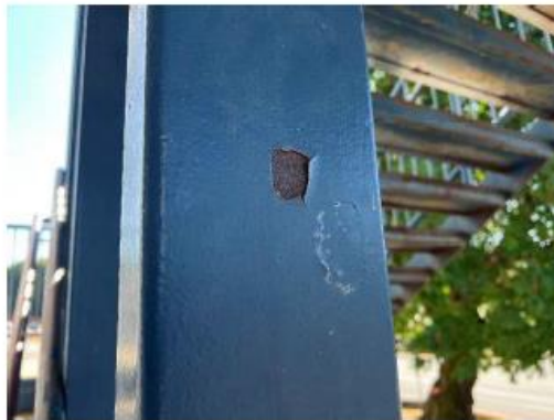
Photo 2 – Damaged paint.
