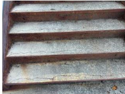
Photo 11 – Corroded steel stair risers.
