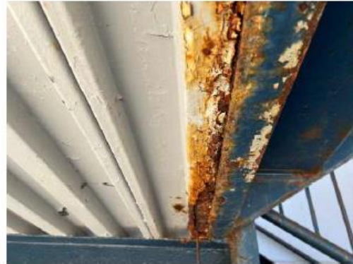
Photo 7 – Corroded steel framing and deck.
