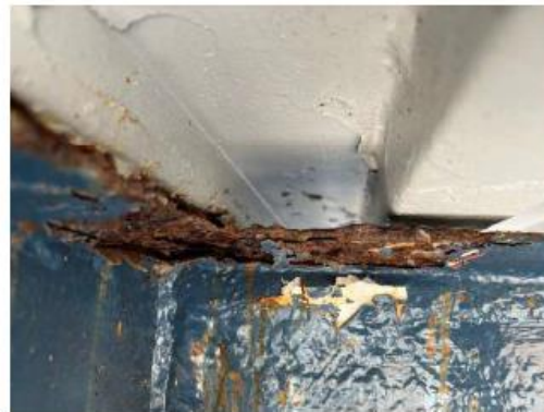
Photo 9 – Corroded steel connection.
