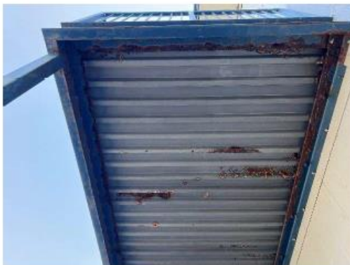
Photo 10 – Targeted steel corrosion.
