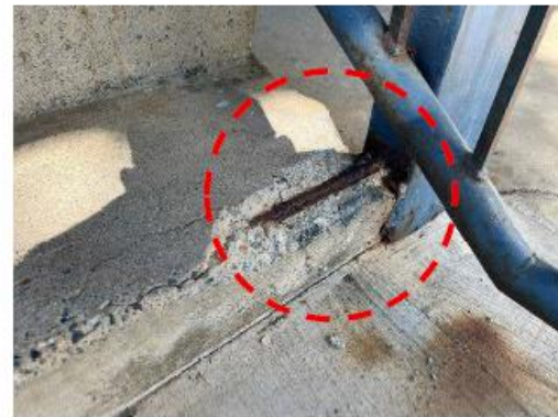
Photo 5 – Delaminated stair nosing.
