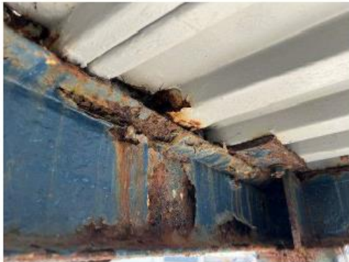
Photo 6 – Advanced steel corrosion.
