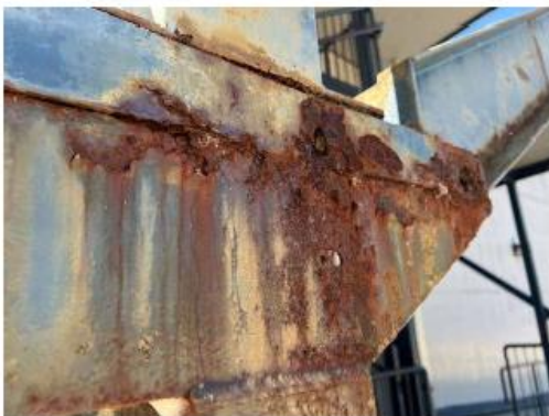
Photo 8 – Advanced steel corrosion.
