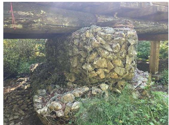
Photo 2: Typical bridge gabion bent.
