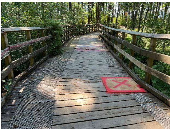
Photo 3: Decking damage.
