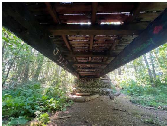
Photo 1: Typical bridge construction.
