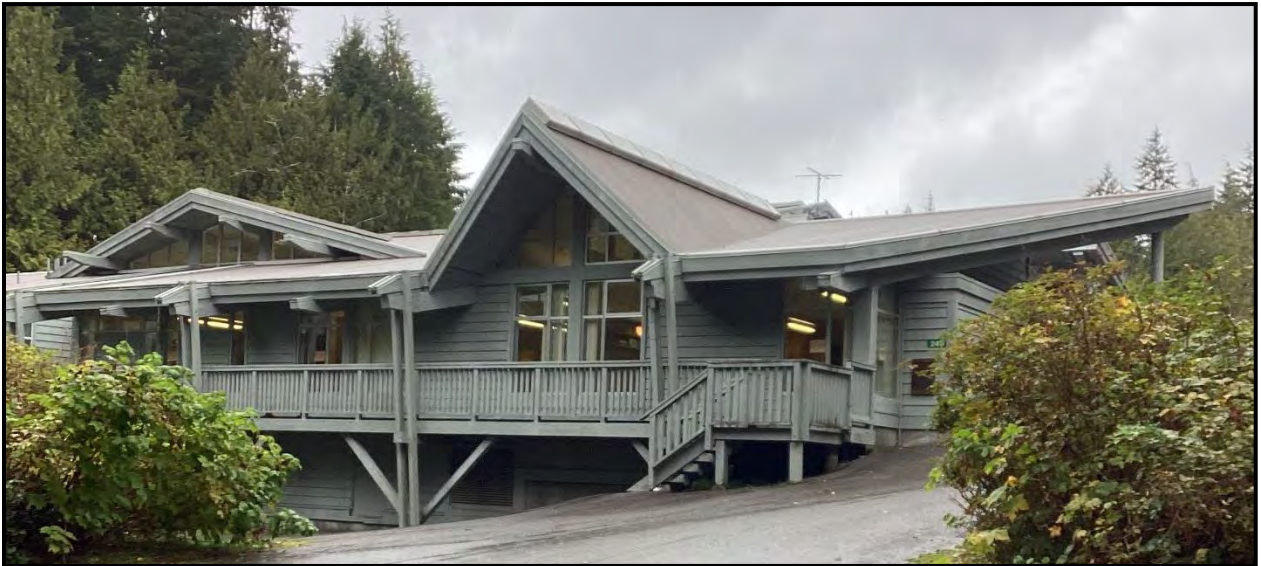
Image 3 – This image illustrates the roof finish, blind-gutters, and exterior siding.
