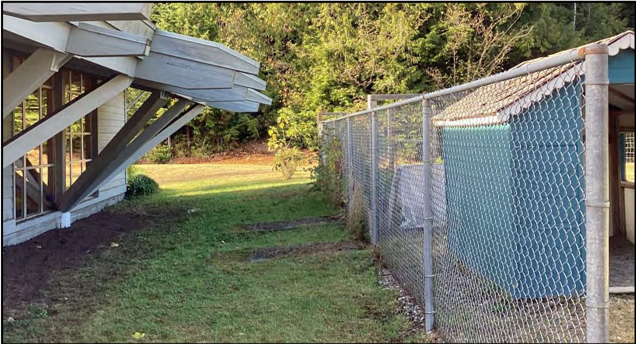
Image 12 - This image illustrates the location of the unmitigated building within Zone 1 near the northeast side of the building.
