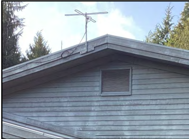
Image 4 - This image illustrates the gable-end venting.
