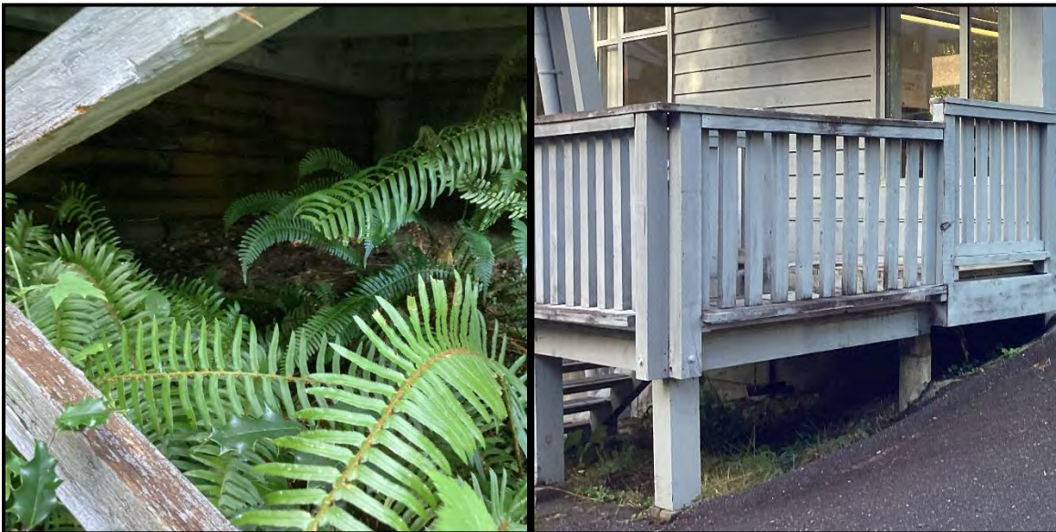
Image 8 & 9 - These images illustrate the surface vegetation growing up under the landings.
