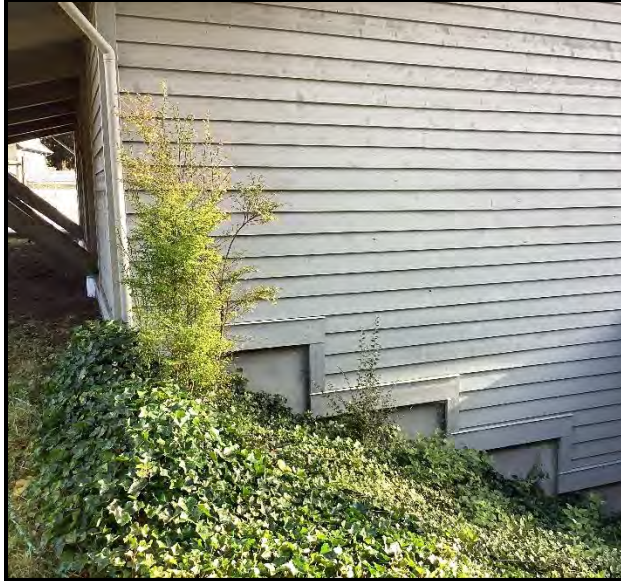
Image 10 – This image illustrates the vegetation growing at the east side and sloped area on the northeast corner of the building.
